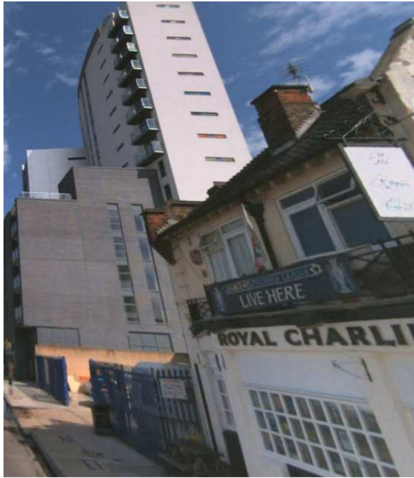
Photo 1: Parkview Apartments – Southern Elevation
