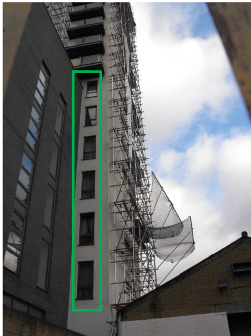
Photo 2: Part West Elevation - Parkview Apartments
