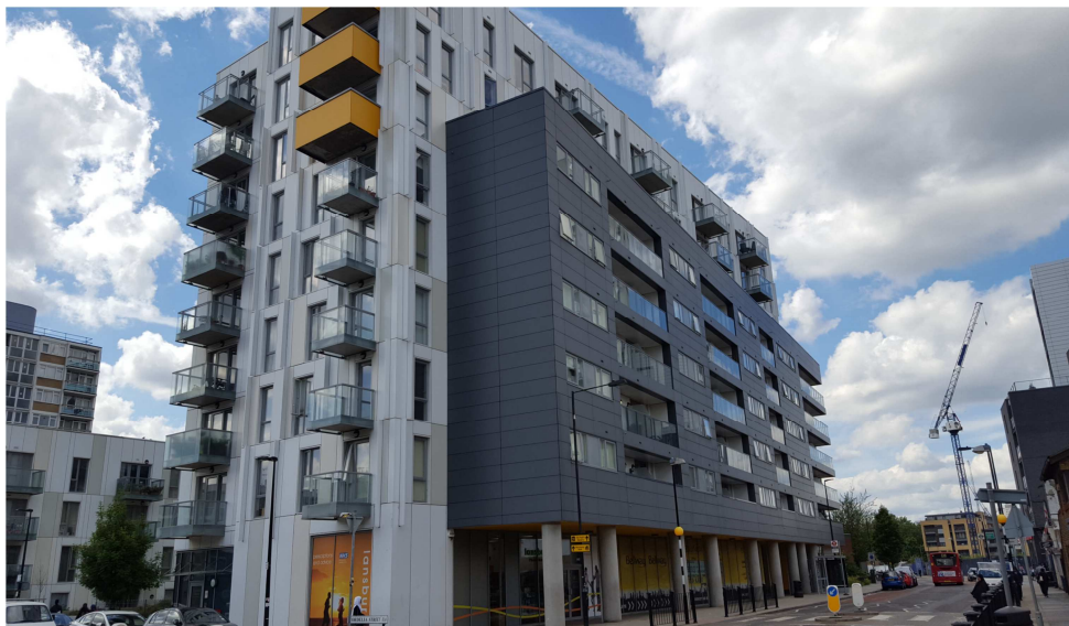
Photo 3: Equinox Building – Chrisp St Elevation
